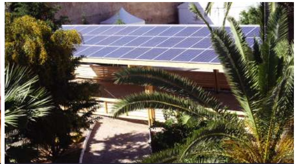
HANGARS AGRICOLES PHOTOVOLTAÏQUE
